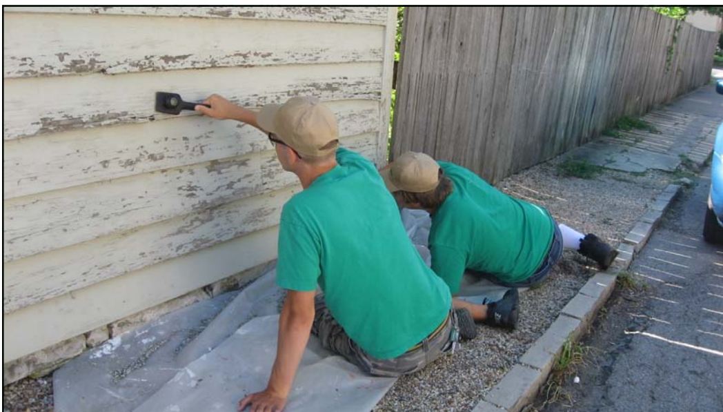
Tom and Huck (of the State Park Youth Corps) scrape and paint a fence at Felix Valle House State Historic Site in Ste. Genevieve.
